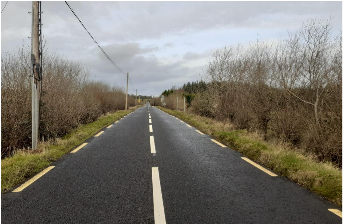
Plate 6.20: Hedging along R314 is generally low, with willow frequent as well as hawthorn and blackthorn. Grassy verges are well represented along both sides of the road. View is from near St. Patrick's College (February 2024).
