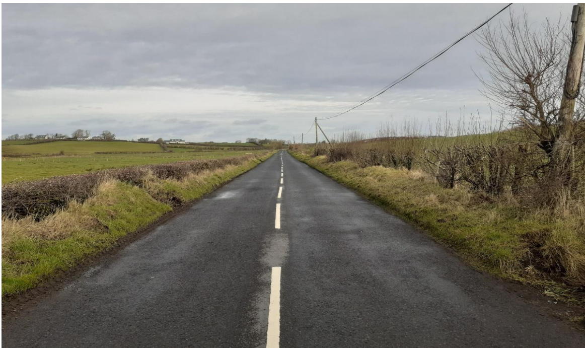
Plate 6.21: View of local road showing low, maintained hedging and grassy banks. Location is at Magherabrack (February 2024).
